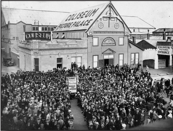
MH 94 | Coliseum Grenville Street Ballarat
